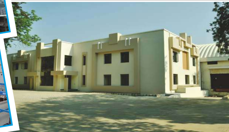
Photographs of a few Manufacturing Units
